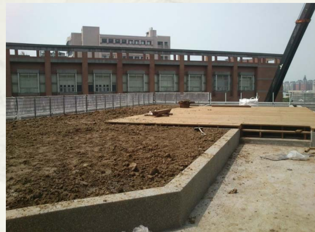
5FL露臺花台沃土回填
