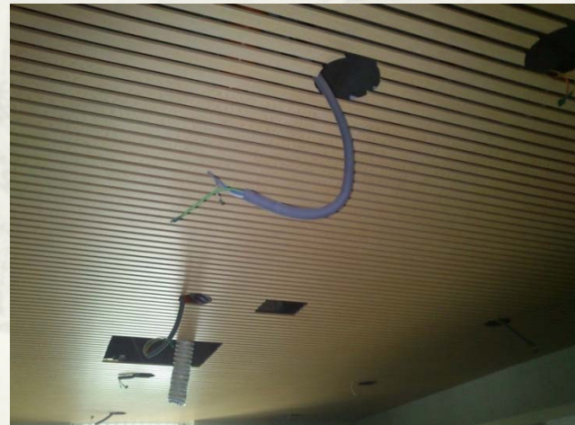
鋁板天花施作
